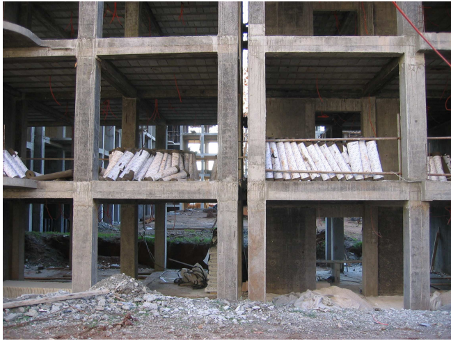
Figure 5.29 c). Joint sismique.
