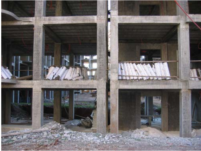
Figure 5.29 c). Joint sismique.
