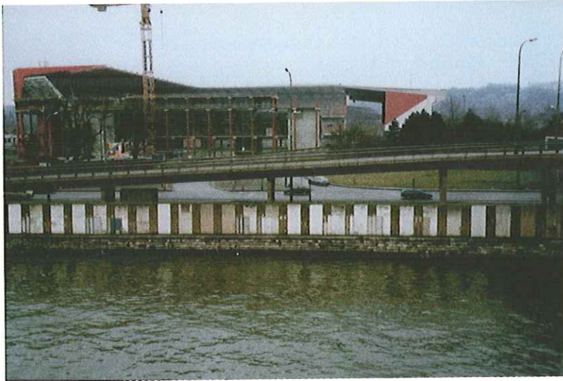
Photo 1: Situation of sandblasted concrete supports
