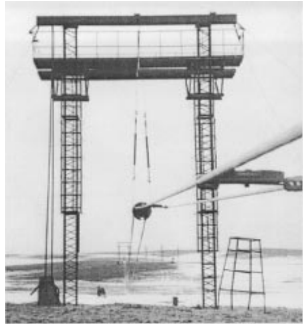
Fig. 1. Southern suspension tower B; Northern (C) is similar.
