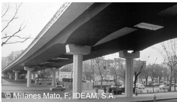
a) Puente de Juan Bravo, Madrid, 1970 (depth-to-span ratio L/h = 40 , weathering steel).
