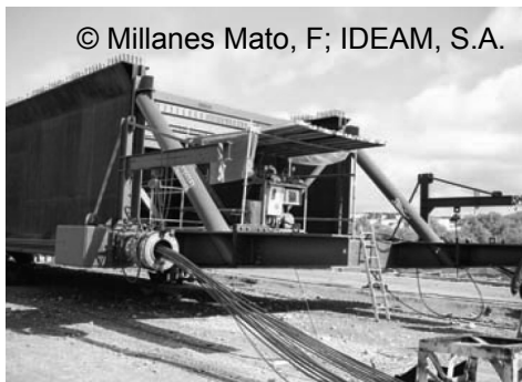
b) Detail of the auxiliary launching structure and the launching cables and jacks.
