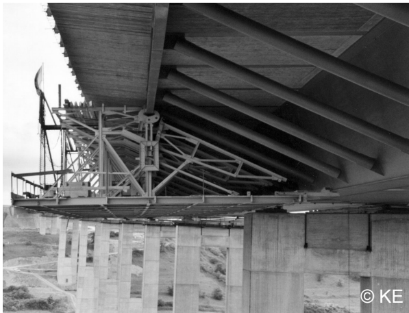
Figure 2-39: Foldable formwork panels, valley bridge Schwarza, Germany, 2002.
