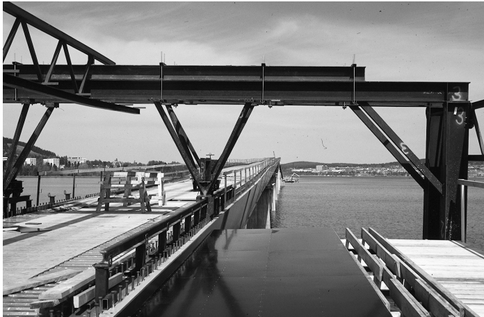
Figure 2-71: Casting of the concrete deck of the Vallundet bridge, Sweden.
