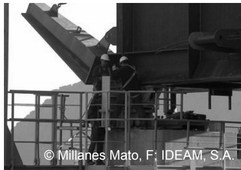
c) Operations during pier passing and nose beam raising.
