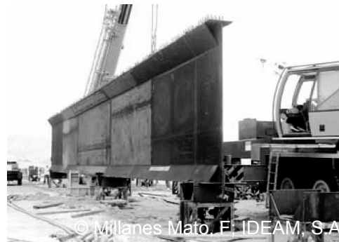
b) Girder with external triangular cells.
