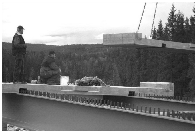
Figure 2-65: Bridge deck element being lifted in place.
