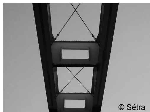
Figure 6-6: Railway twin-girder bridge (TGV Est, Pont à Mousson), France.
