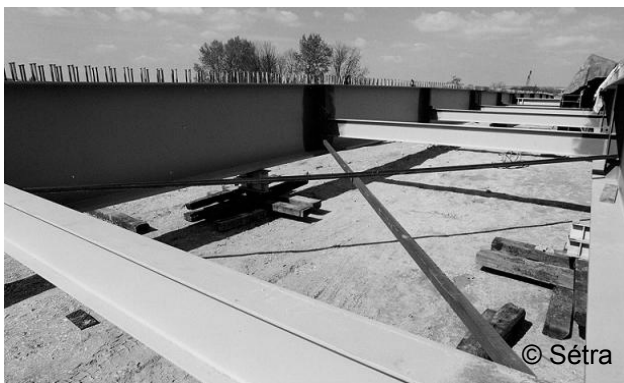
Figure 6-5: Twin-girder bridge in Sens, France.
