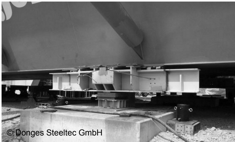
Figure 7-6: Balancer of the valley bridge Elben near Siegen, Germany, 2005.
