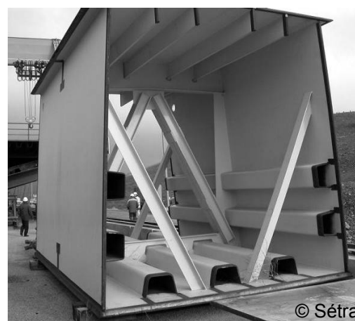
Figure 4-3: Box-girder with closed stiffeners, Millau viaduct, France.
