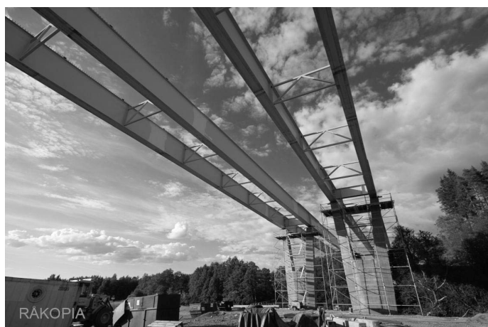
Figure 2-61: Bridge at Rångedala, Sweden, during erection.
