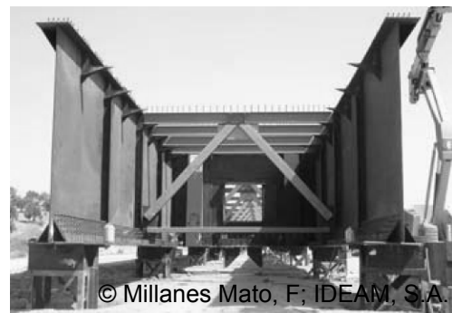
Figure 6-2: Cross bracing as a full lattice.
