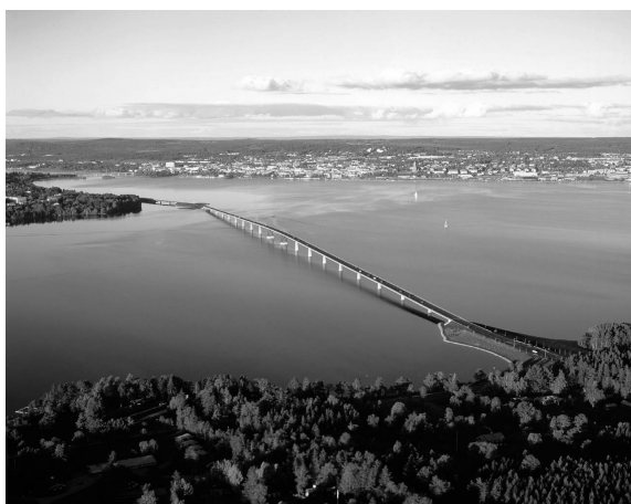
Figure 2-70: View of the Vallsundet bridge, Sweden, and the triangular supports over the navigation channel.
