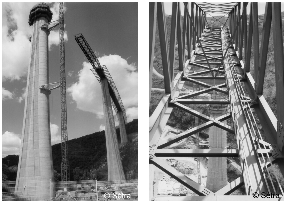
Figure 7-9: Launching nose for the Verrières viaduct near Millau, France, 2002.
