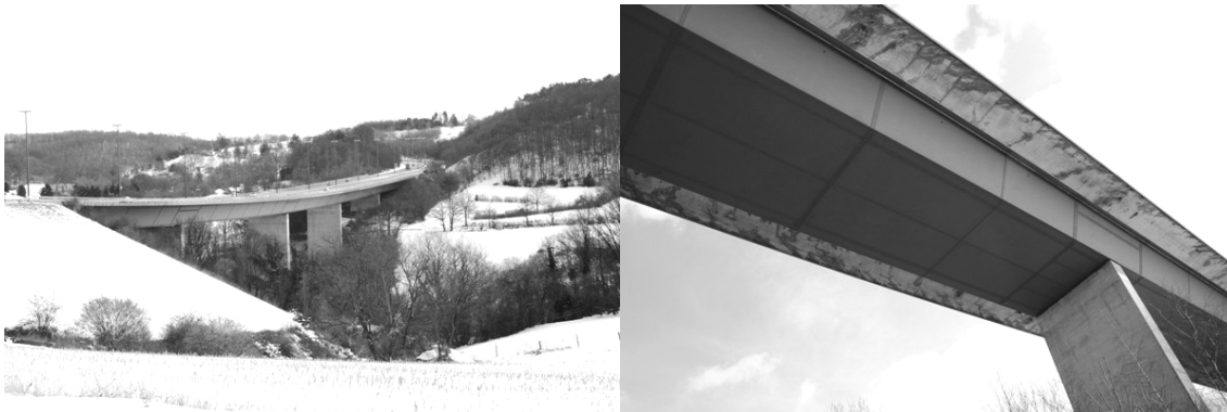
Figure 2-16: The viaduct of Polleur, Belgium.
