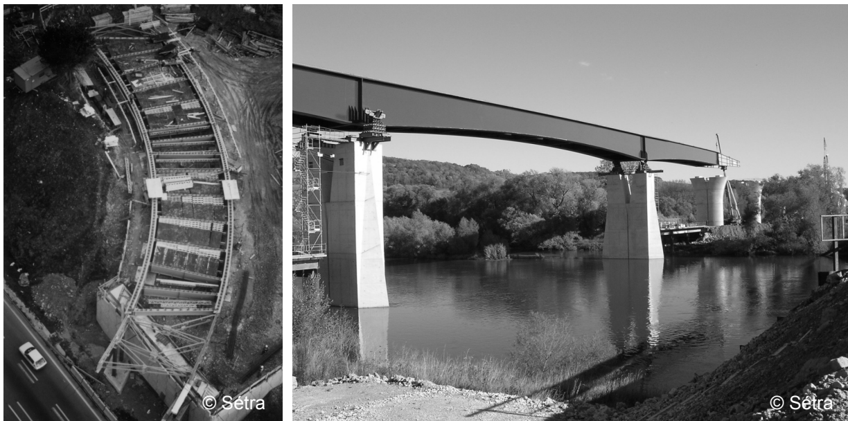
a) Launching of a curved bridge near Cannes, France.
