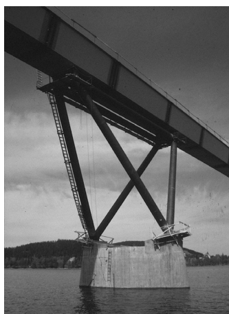
Figure 2-70: View of the Vallsundet bridge, Sweden, and the triangular supports over the navigation channel.
