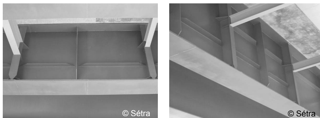
Figure 5-6: Twin-girder bridge in Triel-sur-Seine, France, 2003.
