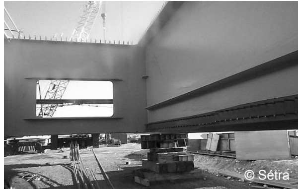
Figure 6-4: Railway twin-girder bridge (TGV Est, Canal de l'Ourcq) with diaphragms, France, 2006.
