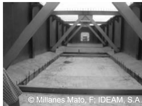
d) Prefabricated slabs and on site concrete in the bottom flanges.
