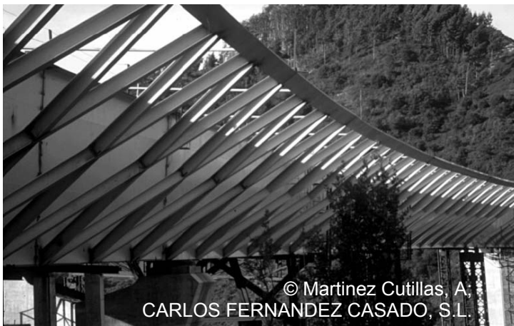
Figure 2-54: The viaduct of Tina Menor, lateral truss [56].
