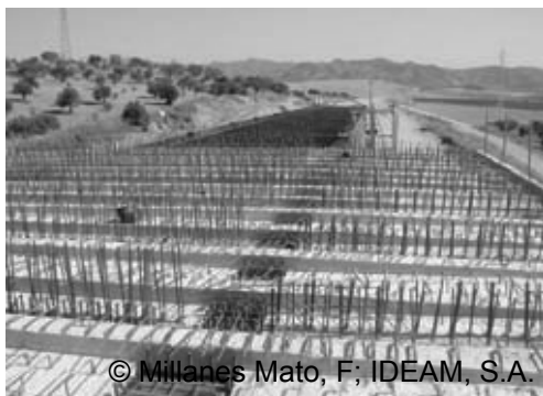
c) Prefabricated slabs in the top flange.
