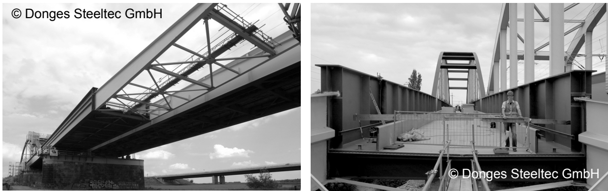
Figure 5-12: Launching of a railway bridge near Riesa, Germany, 2005.
