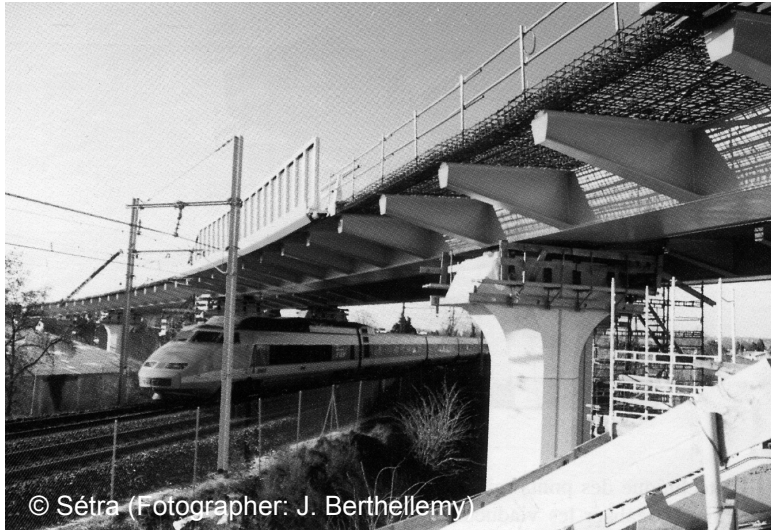
Figure 7-10: Croix Verte viaduct, launching above train lines, Avignon, France, 1994.
