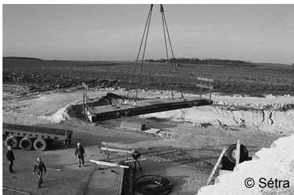
Figure 2-22: Use of prefabricated slab segments.
