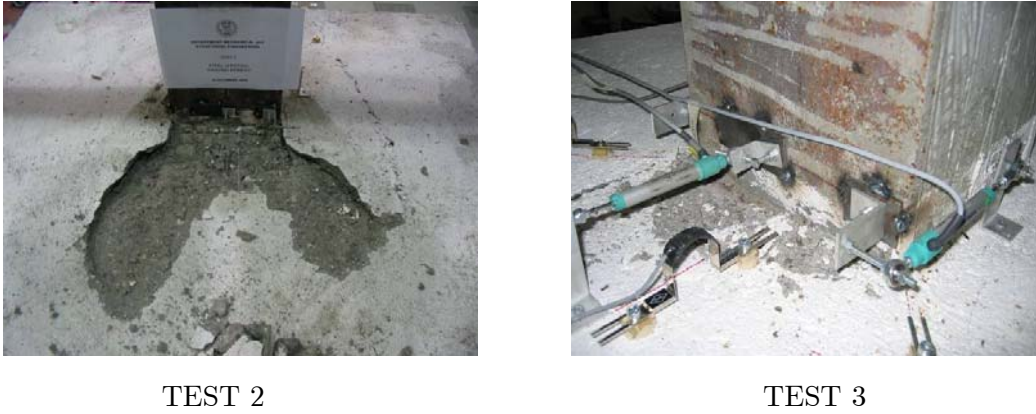
Figure II.26. Crushing of the concrete in front of the column at the end of TEST 2 & 3
