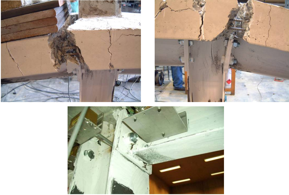
Figure III.52. External composite joints at the end of the test
