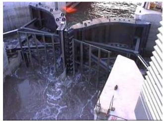
Fig.6 - Vertical-axis sector gates
