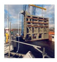
Fig. 4 -Mitre gates supported only at their top hinges
