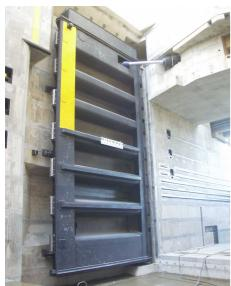
Fig. 2 - Folded plate of a mitre gate at Uelzen II
