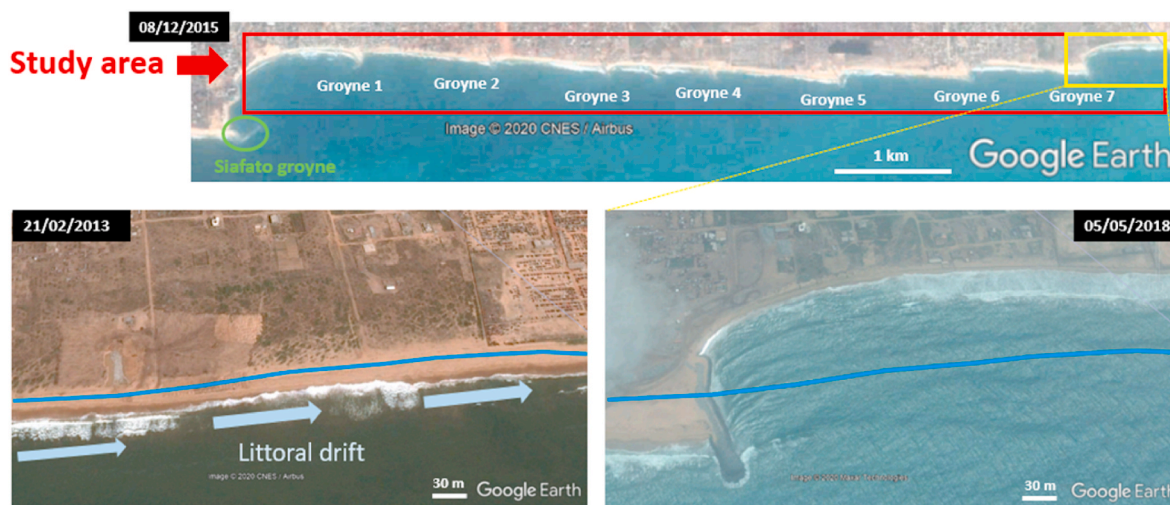
Fig. 4. Rapid erosion in the east of the protected zone.
