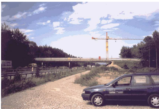
Figure 5: View of Z24 bridge.
