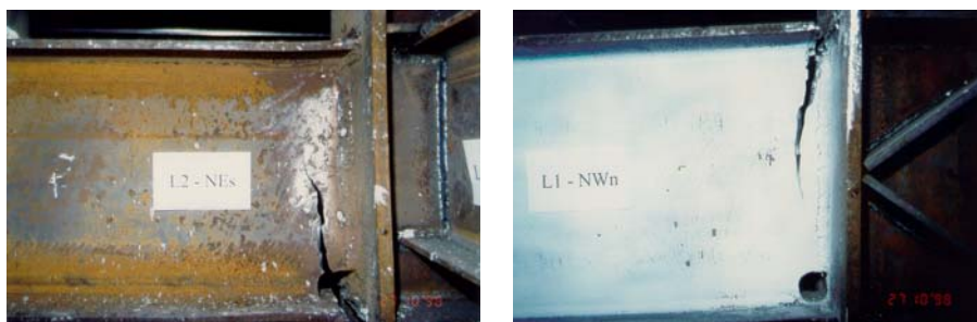
Figure 4. Cracks
