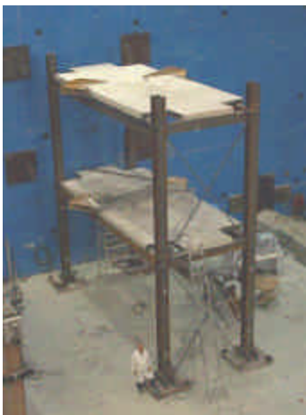
Fig. 1: View of the Steel-Quake structure
