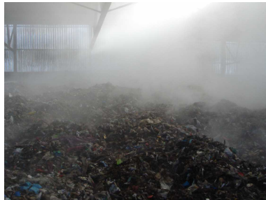
Installation de compostage
