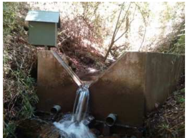
Figure 1. V-notch weir (sediment trap) at the outlet of the catchments
