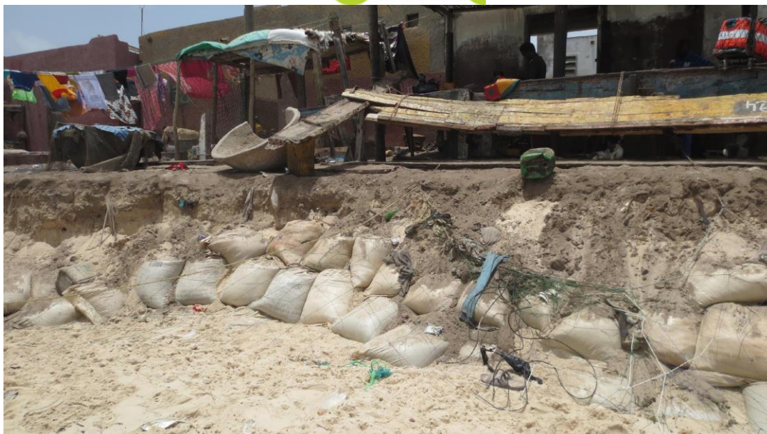
Figure 27 - Sand bag barriers stabilized with old fish netting. Goxum Bacc, Saint-Louis, Senegal.
