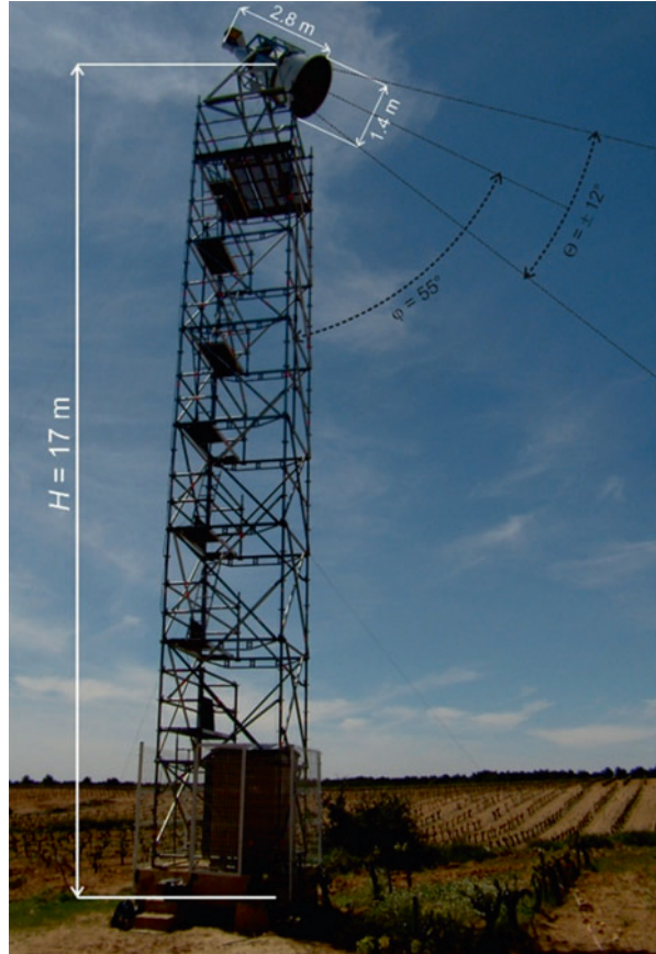
Fig. 2 L-band radiometer ELBARA II mounted on a tower at the MELBEX III site in Spain used for the calibration and validation of Soil Moisture and Ocean Salinity (SMOS) satellite observations
