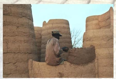
Cob, the earth built in layers
