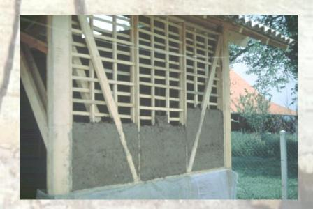
Wattle and daub, the earth used in filling loadbearing structures, usually made of wood.
