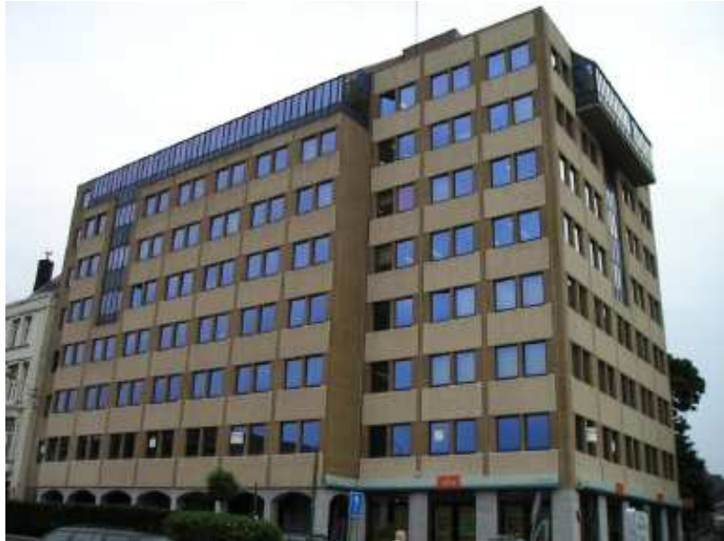
Figure 1: building of interest
