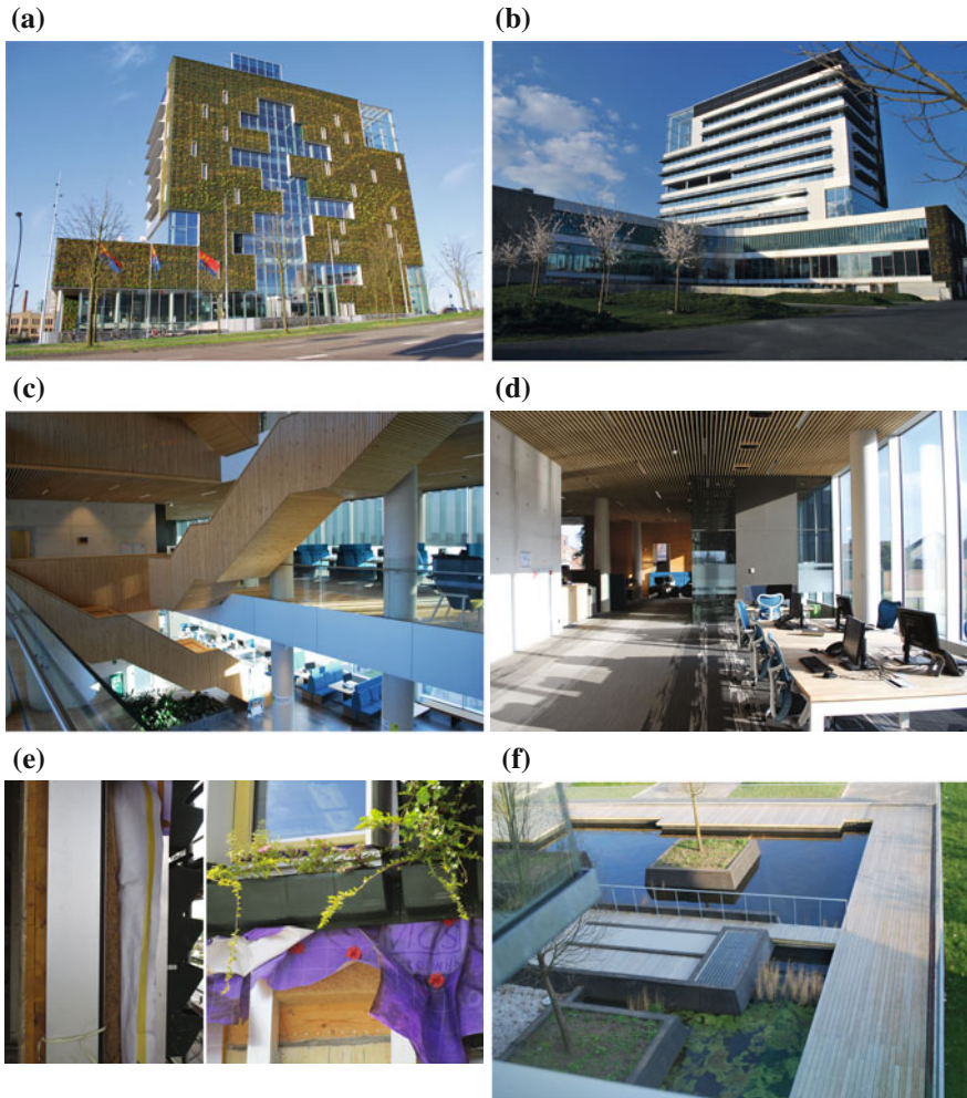
Fig. 6.3 a Overall view of the Green Façade (Biosphere), Venlo City Hall, Venlo, The Netherlands. b Overall view of the South Façade (Technosphere) with solar protection. c The void crossing the building centrally and providing natural lighting in connection to the solar chimney. d Office spaces and flexible working areas. e Cross section in the Green Façade showing the different wall layers and construction system. f The hylofilter is a natural wastewater treatment pond using biological and bacteriological purification techniques
