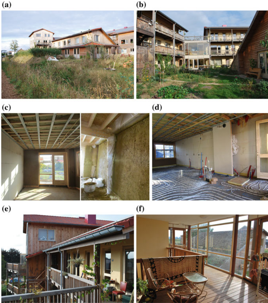
Fig. 6.4 a Overview of Iewan Social Housing Project, Lent, The Netherlands. b Internal garden used for permaculture and underground water storage. c Straw and loam construction and lime sandstone. d Under floor heating is coupled to a biomass heating system. e Southern façade terraces provide solar protection during summer and view and circulation for tenants. f Winter terrace space for tenants
