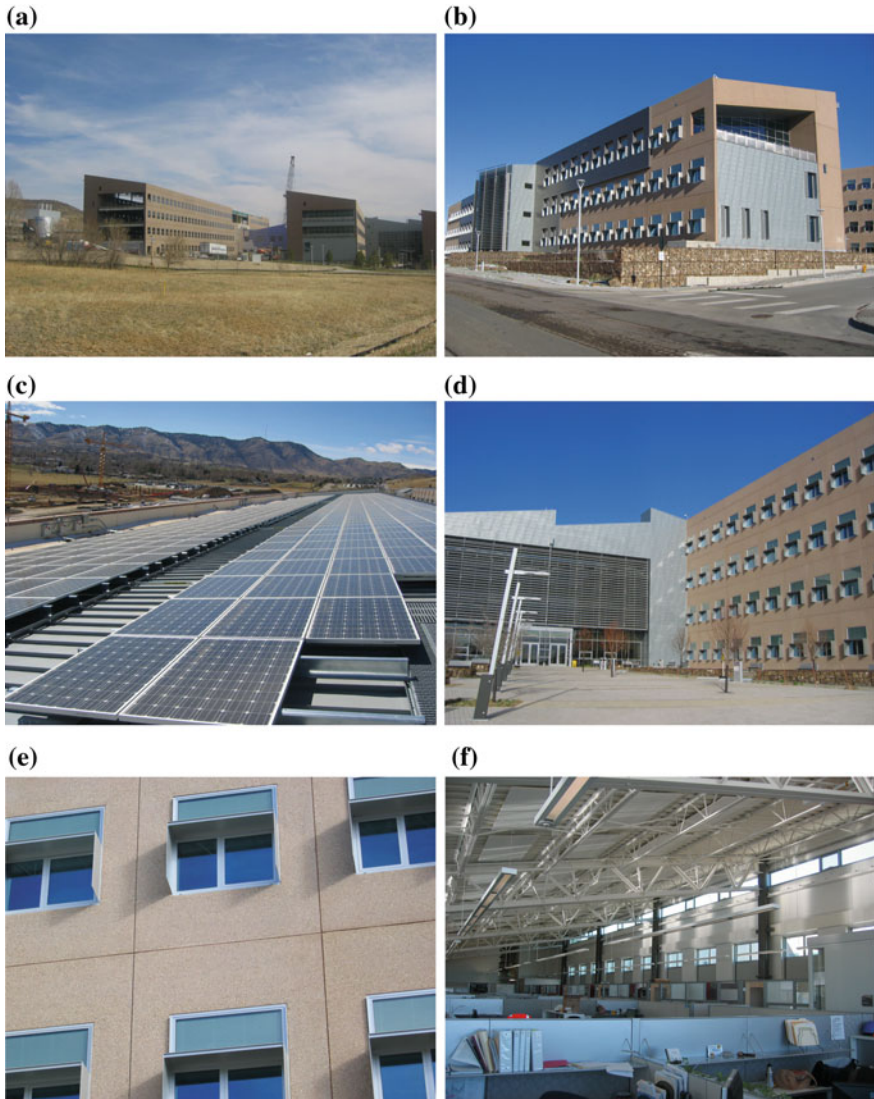
Fig. 6.1 a Two wings optimized to allow natural lighting and ventilation, RSF, NREL, Golden, Colorado, US. b The South Wing is optimized for a window-to-wall-ratio of 25% and the east glazing surface is minimized. c PV array of mono-crystalline panels of 17% efficiency. d The South Wing is optimized for a window-to-wall-ratio of 25% and the east glazing surface is minimized. e Windows design was optimized to reduce the effective view glass and provide solar protection. f The open space office was optimized for maximum natural lighting and natural cross ventilation
