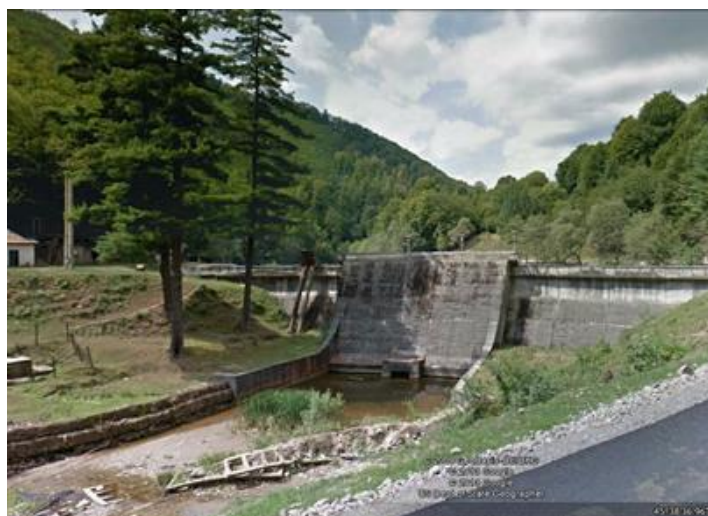
Figure 1. Sadu II Dam, Sibiu, Romania, the oldest dam in Romania Source: Google Earth
