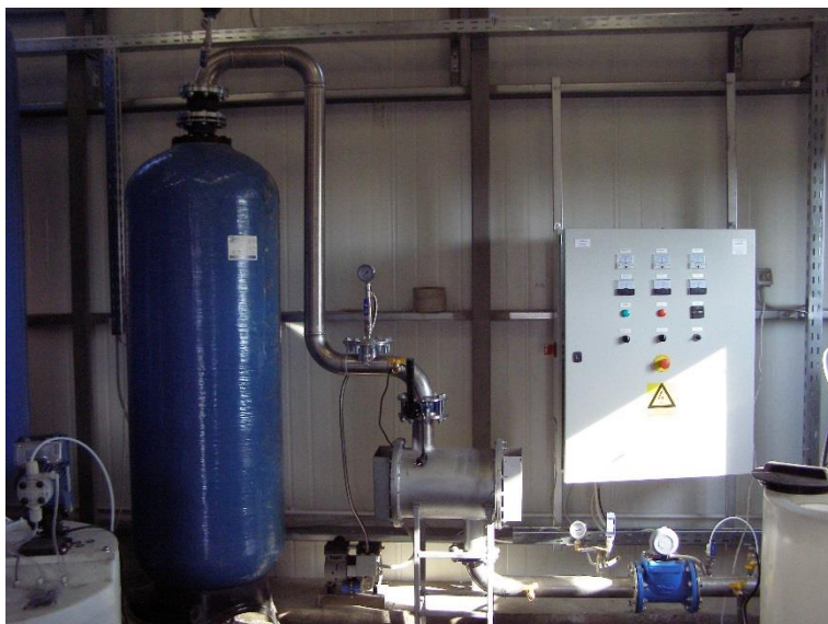
Figure 2. Electrochemical step (pre-oxidation) in MAPOx-20 module from drinking water station Cruset, Gorj county
