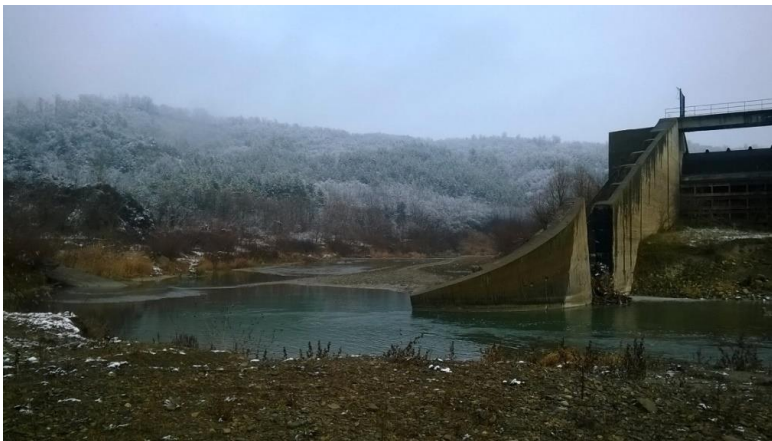
Figure 3. The left bank of the Belci dam
