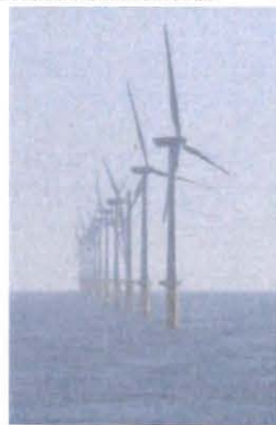
Figure 1 Steel monopile offshore wind turbines.
