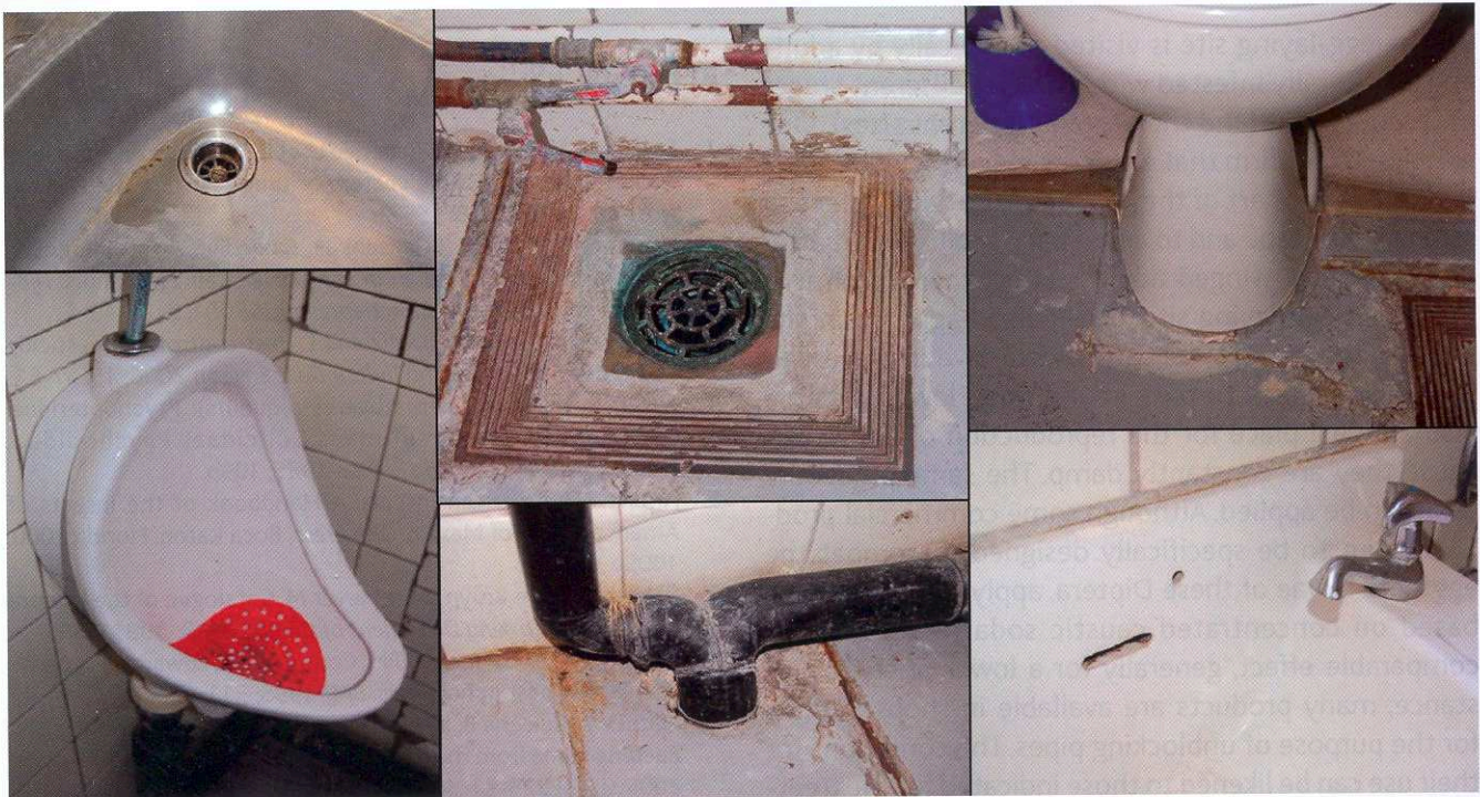
Figure 3. Risk areas which can serve as an egg-laying site for adult "mothflies".
