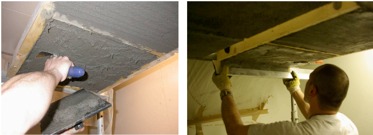
Fig. 4 : Application of mortars on concrete substrate and finishing operations
