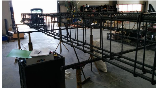
Figure C-1. Assembled reinforced cage of the beam
