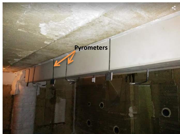
The view of the beam from inside the furnace
