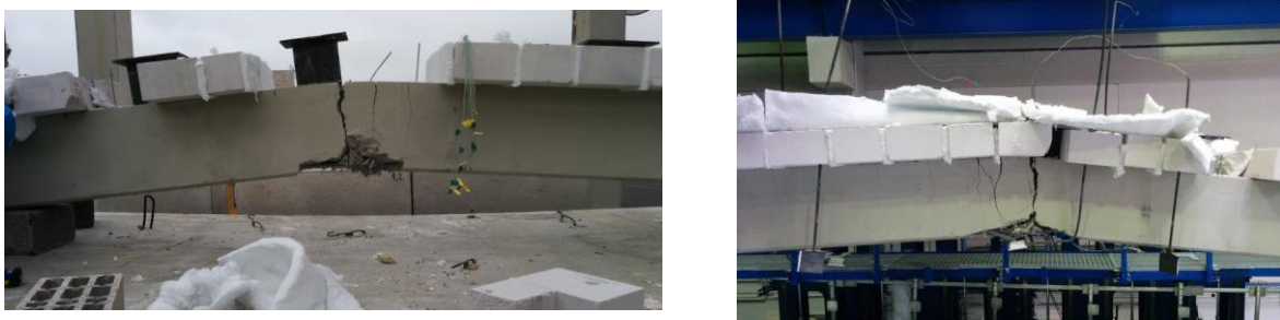
Figure 6-58. The failure mode of the beam in the TEST 3
