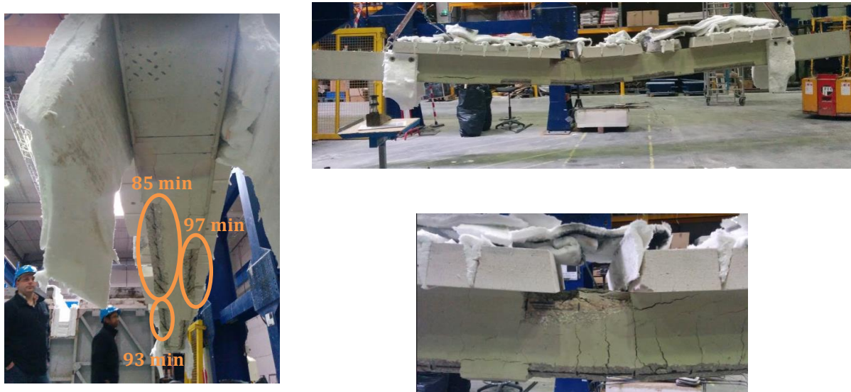
Figure 6-27. The beam after the fire exposure.
