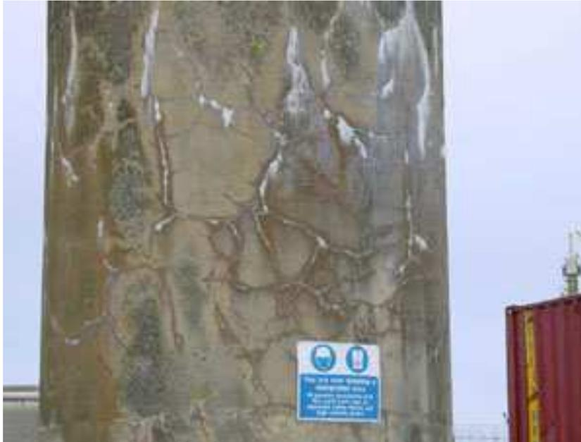
*Harbour installation from the 1970's containing Diorite and granites with opaline veining coarse and fine aggregate (BRE-UK).*
