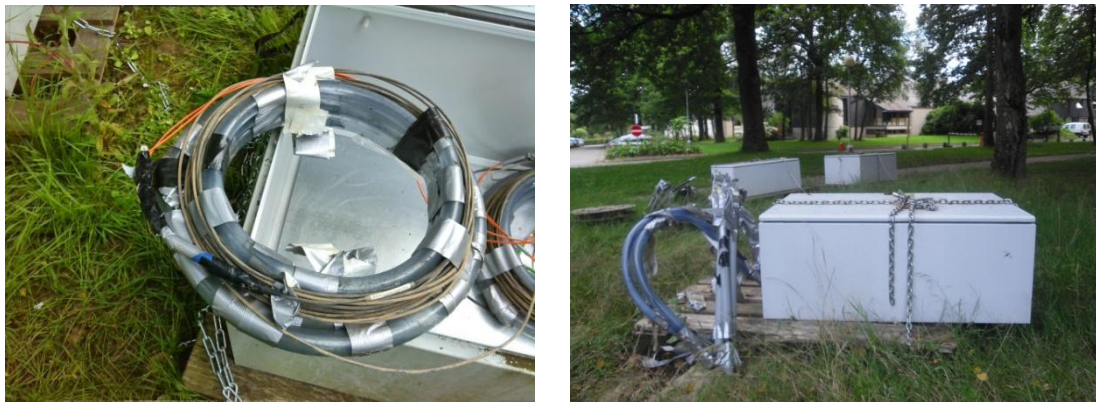
Figure 6.4 - Fiber optic cable loops (left) and protection metallic box (100 cm x 60 cm x 40 cm) (right)
