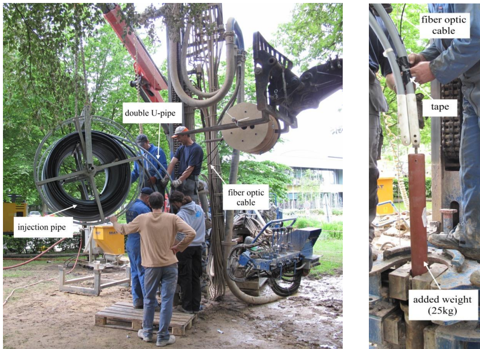
Figure 2.4 - Geothermal double U-pipe and fiber optic cable installation
