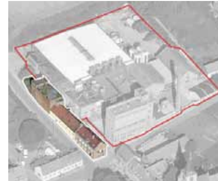
Aerial view of site. © bing.com/maps
