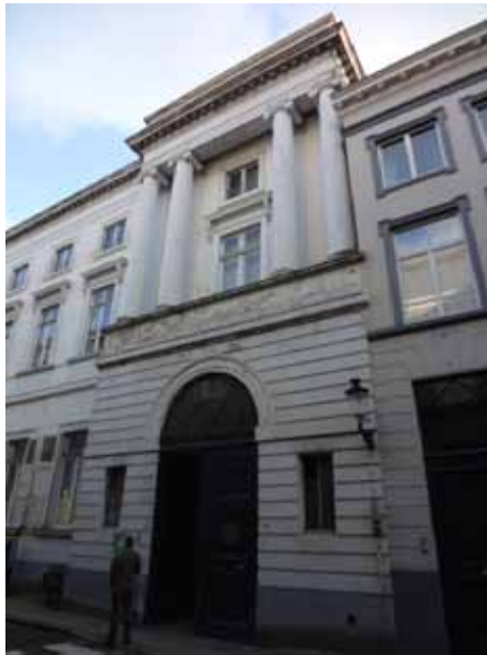
Facade of House de Nieulant in the Sint-Jansstraat © E. Bouton
