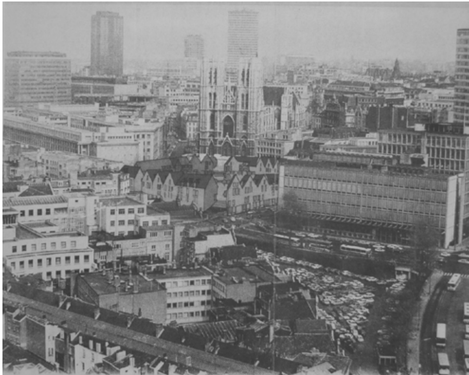
Photographic montage showing the project of a new building block in front of Brussels cathedral, ca 1979 © KULeuven, Lemaire archive
