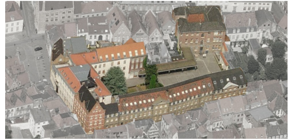
The Hemelsdaele School Complex in Bruges © Bing Maps
