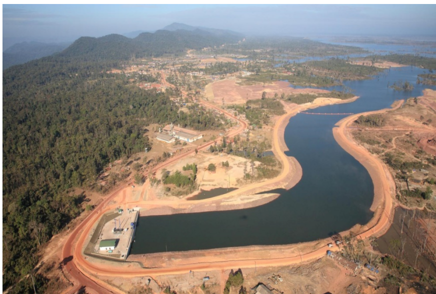
Photo 3: Headrace Channel with the Location of the Water Flow Intake of the Headrace Tunnel.
