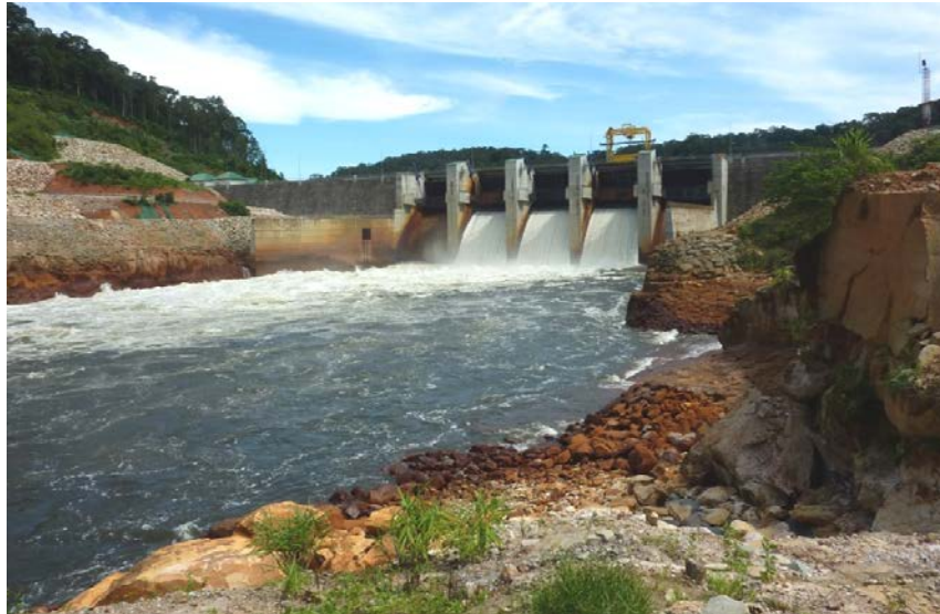
Photo 2: The Nakai Dam with Spillways on the Nam Theun at Keng None
