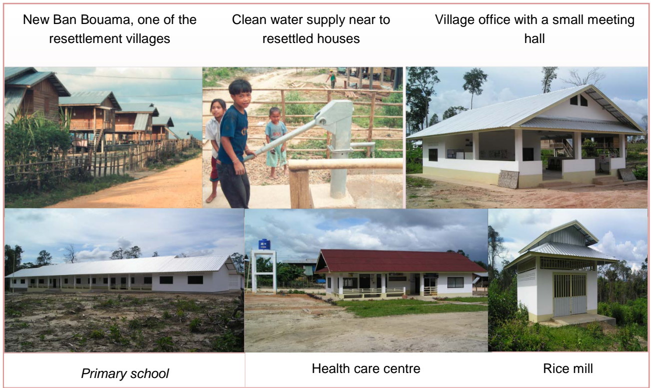
Photo 8: Infrastructure of the Resettled Village Provided by the Project
