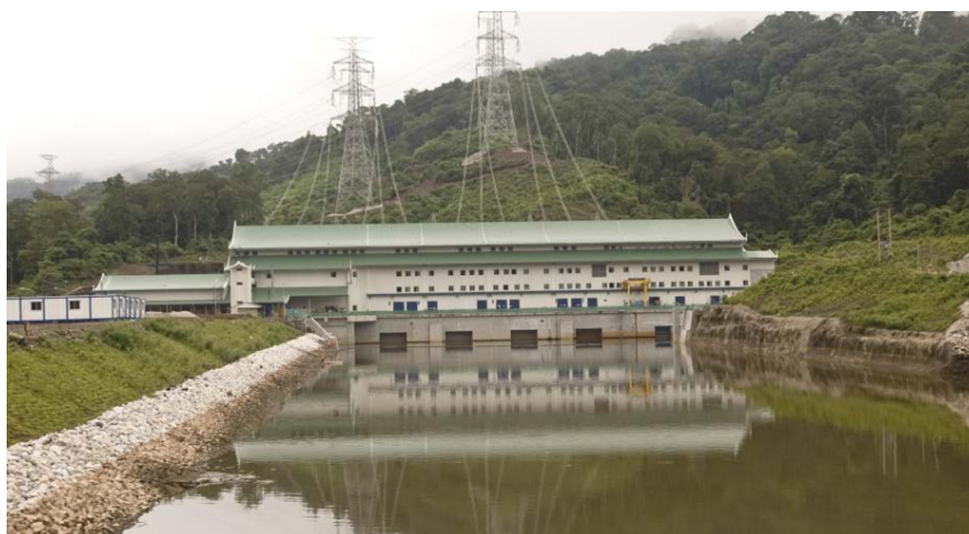
Photo 4: The Nam Theun 2 Power Station, Viewed from the Tailrace Channel.
