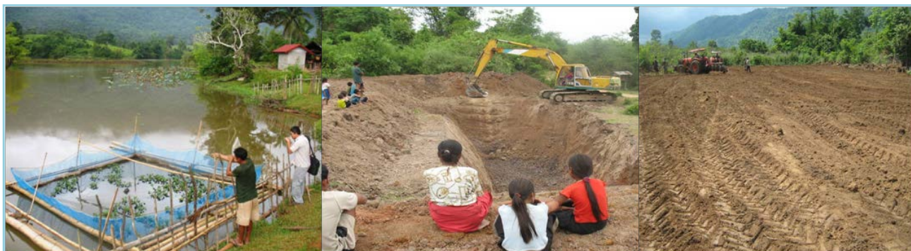
Photo 16: Livelihood Restoration Programme Downstream of the Nakai Dam, Khamkeut District
