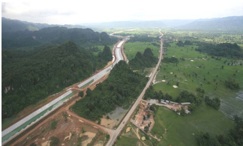
Photo 5: View of the 27 km Man-made Channel Flowing Down from the Powerhouse/Regulating Dam to the Xe Bang Fai
