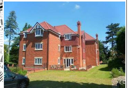
Figure D: Low-rise apartment block
