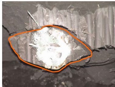
Figure 6.43: Eye-shape fractures around a resin-immobilized borehole [Blümling et al., 2007].
