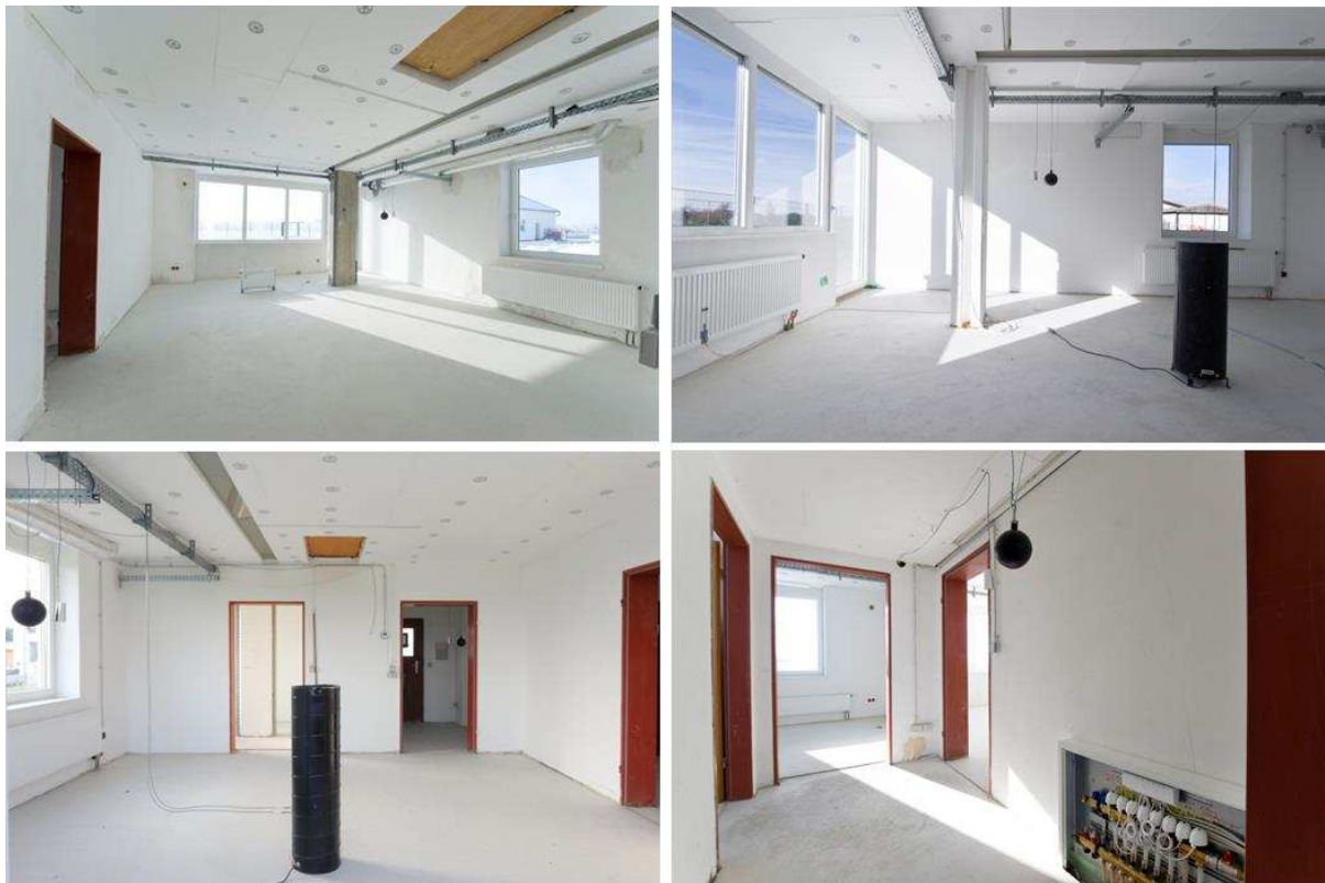
Figure 7: Internal views of the Twin Houses.
