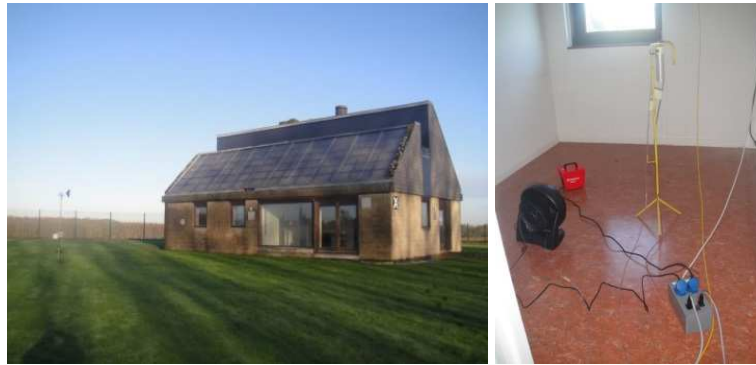
Figure 8: Localization and plans (upper), general outside view and inside view of a zone (lower) of the BBRI X2 experimental building
