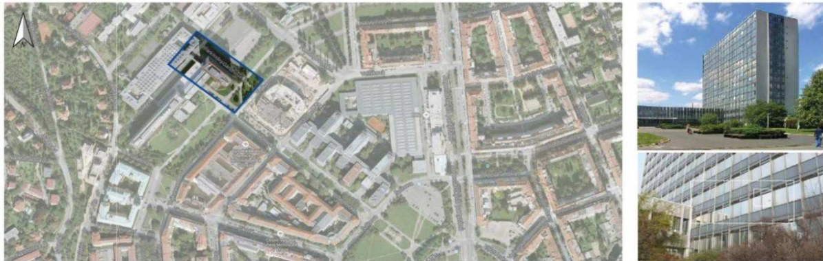
Figure 3: Building's localization and views.
