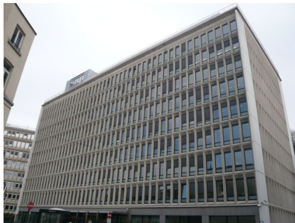
Fig. 3. Case Study Building (SW façade)
