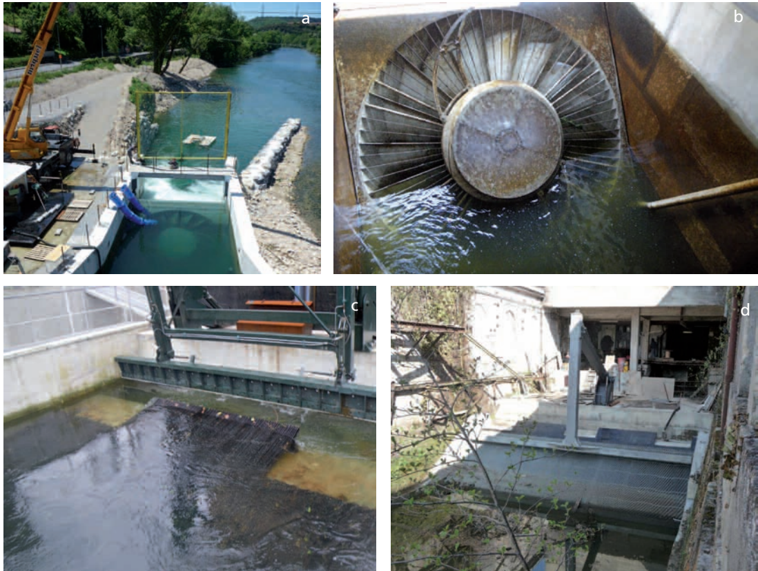
(a, b) Example of a fish-friendly turbo-generator, (c, d) fish-friendly water intake with a rising incline made of narrowly spaced bars and surface bypasses enabling fish to escape downstream.
