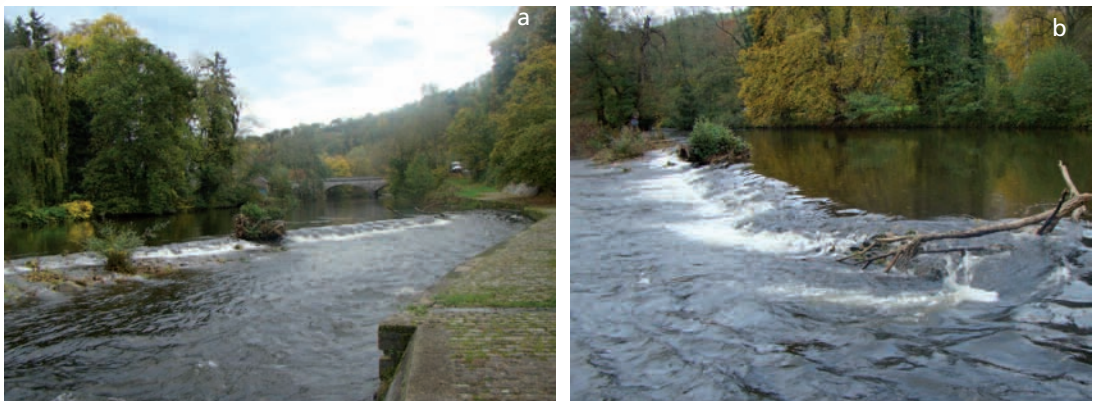
Examples of obstacles cleared by radio-monitored pike in the Ambève River (Southern Belgium). The photos show hydrological conditions lower than the optimum passage discharge. (a) General view of the obstacle, (b) zoom on the passage zone.
