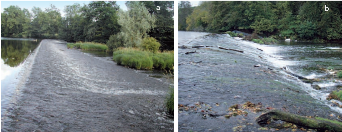
Examples of obstacles that a certain percentage of yellow eels can overcome by crawling. These structures nonetheless hinder the free movement of the species.
