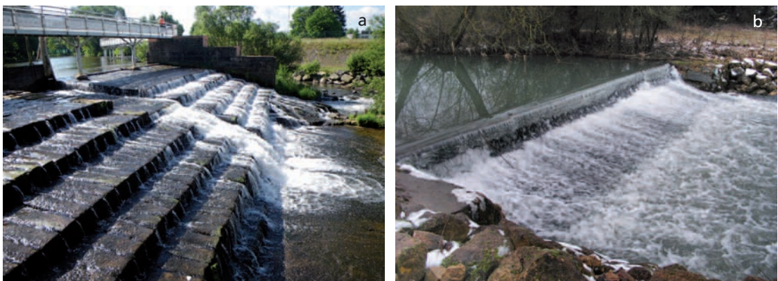
Examples of steps in inclined downstream faces. (a) A stepped weir, (b) a sill on the crest of the weir.
