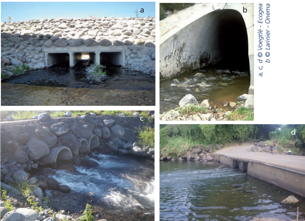
(a) Example of a road structure built with box culverts, (b) example of a structure comprising an apron with some riprap, (c) road structure built with round culverts, (d) road structure built with box culverts.
