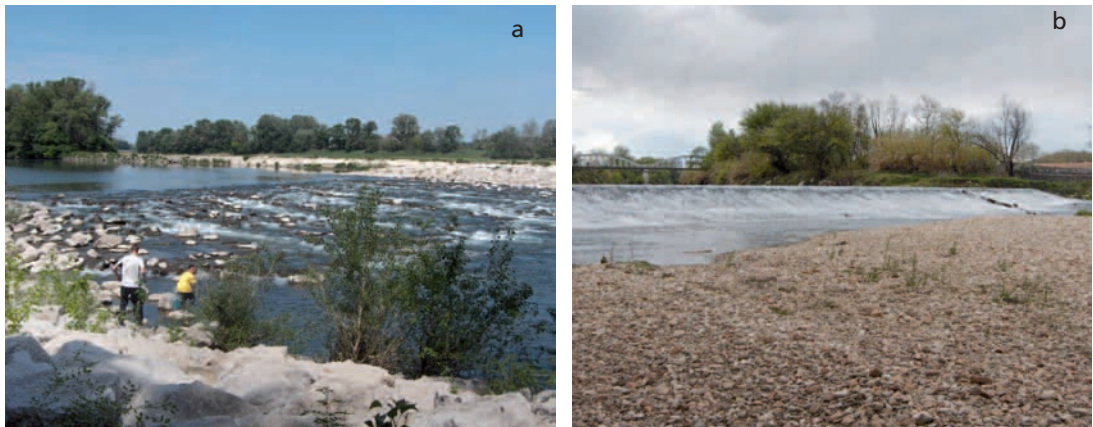
Examples of passable and impassable obstacles for shad. (a) Weir on the Ardèche River that shad can clear. The photo shows hydrological conditions enabling passage. (b) Weir on the Cèze River that shad cannot pass, except when discharges are very high, which is rare during the migratory period.
