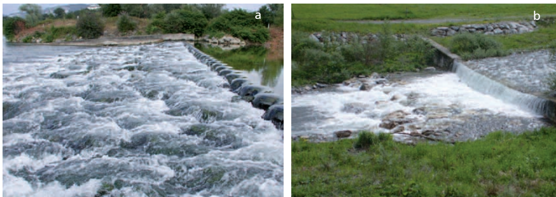
Examples of rock weirs with steps.
