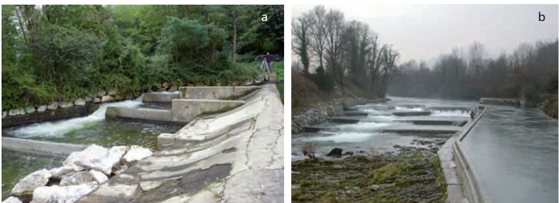
Examples of pre-barrages. (a) Pre-barrages at the Guilhot dam on the Ariège River, (b) pre-barrages at the Gurmençon dam on the Gave d'Aspe River.
