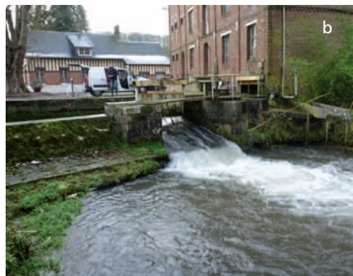
Diagrams and examples of gates under pressure and not under pressure. (a) Photo of a gate under pressure, (b) Photo of a free-surface flow (gate not under pressure).
