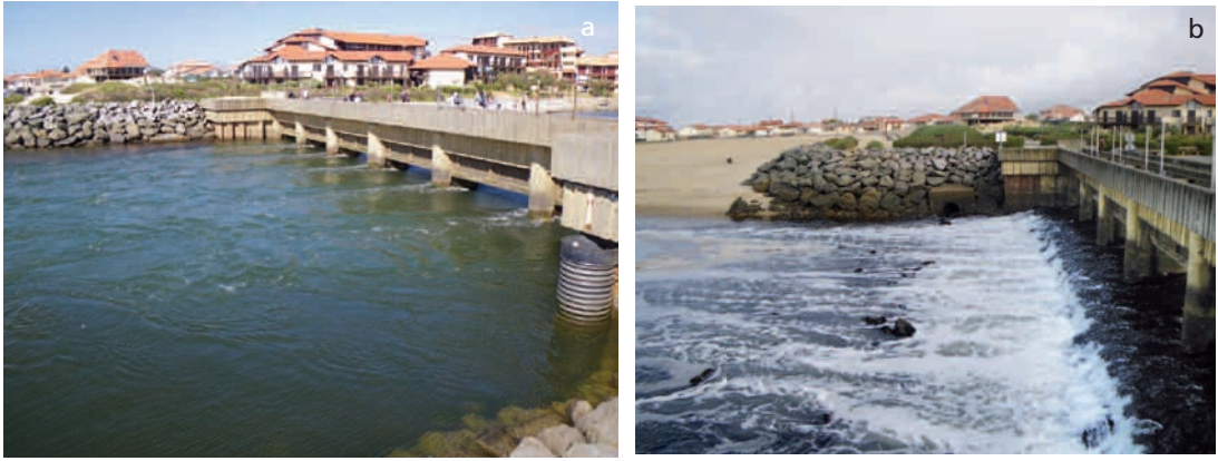
Example of the Lac Marin (on the Courant de Soustons River in the Landes region, SW France). (a) High tide, the sea water flows over the obstacle into the lake upstream, (b) at low tide, a weir maintains the water level in the lake.
