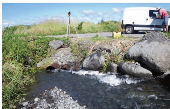
Example of high flow velocities created upstream of culverts.
