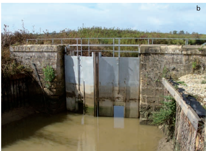
Examples of orifices created to allow the passage of fish. (a) and (b) Orifices positioned in the lower section of tide gates to allow the passage of fish when open, at Jalles in South-West France.
