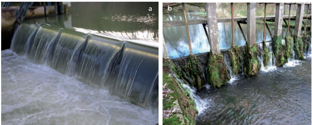
Flows over the moving parts (gates) of weirs. (a) Weir with spillway gates. (b) Weir comprising a series of lift gates.
