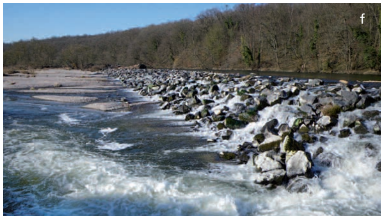
Examples of fixed weirs. (a) Vertical weir, (b) weir with numerous steps, (c) inclined weir with a step at the top, (d) inclined weir, (e) rock chute (rock weir with a slight slope), (f) rock weir with a steep slope.
