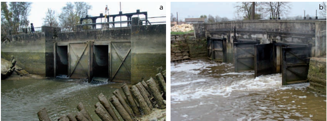
Examples of tide gates. (a) Tide gates at the outlet of the Arcins marshes in the Gironde department, SW France. (b) Tide gates on the Livenne River.
