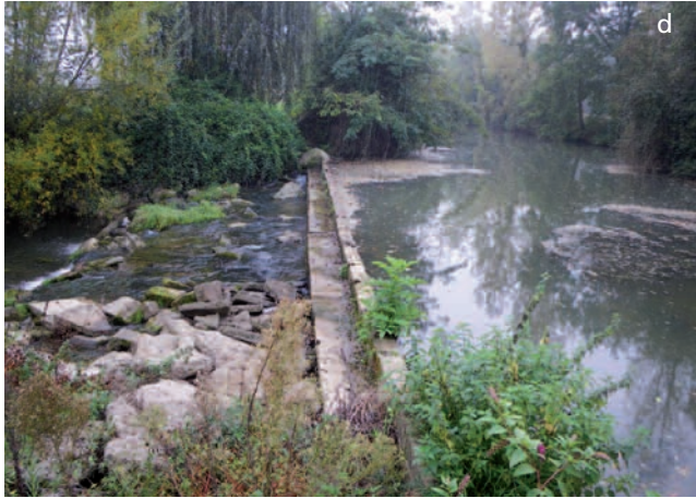
(c) (d) Examples of riprap used to protect the foundation of a weir from erosion.
