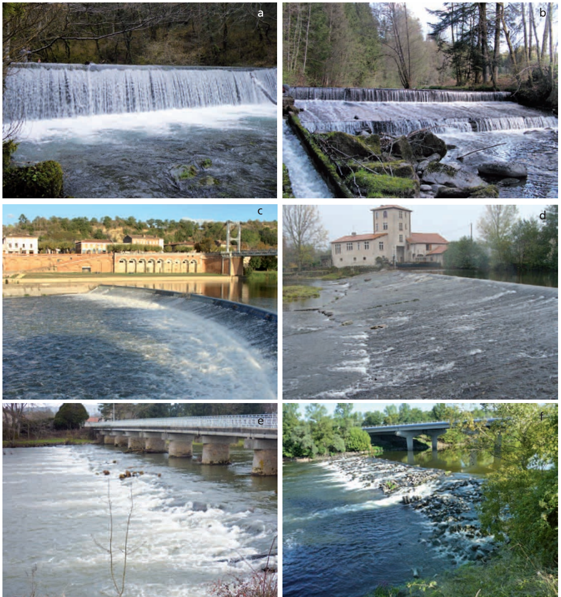
Examples of obstacle configurations often encountered. (a) Vertical weir with a plunging jet, (b) complex weir with an upstream step, a glacis and a downstream waterfall, (c) inclined weir with a step at the top, (d) inclined weir, (e) rock weir, (f) rock weir with a steep slope under low-flow conditions.
