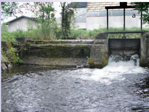
Diagrams and examples of gates under pressure and not under pressure. (a) Photo of a gate under pressure, (b) Photo of a free-surface flow (gate not under pressure).
