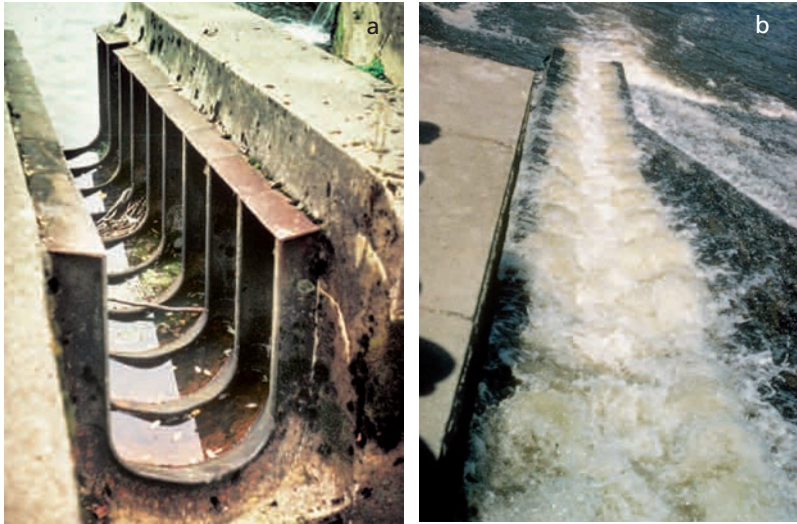
Examples of fish passes with Fatou baffles. (a) Fish pass with Fatou baffles at Halsou on the Nive River, (b) idem at the Claies de Vire site on the Vire River.
