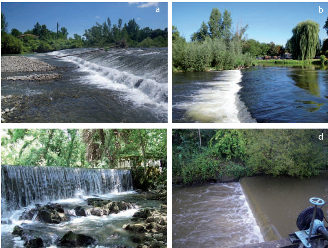
Examples of plunge pools at the foot of obstacles. (a) and (c) Insufficient pools, (b) and (d) sufficient pools.
