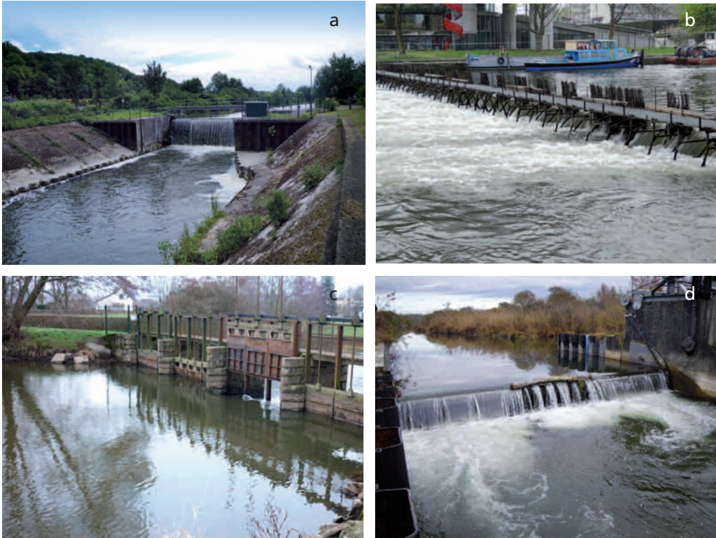
Examples of movable weirs. (a) Weir equipped with a lift gate allowing flow both over and under the gate (La Vilette weir at Louviers on the Eure River), (b) needle weir (Robertsau weir in Strasbourg on the Ill River), (c) weir comprising several lift gates (gate system at the Autun camp grounds on the Ternin River), (d) weir equipped with a spillway gate (Probert weir on the Sainte-Eulalie River).
