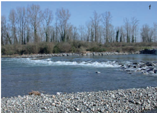
e) (f) Examples of stabilisation weirs for the riverbed of the Gave de Pau River, designed to avoid downcutting.
