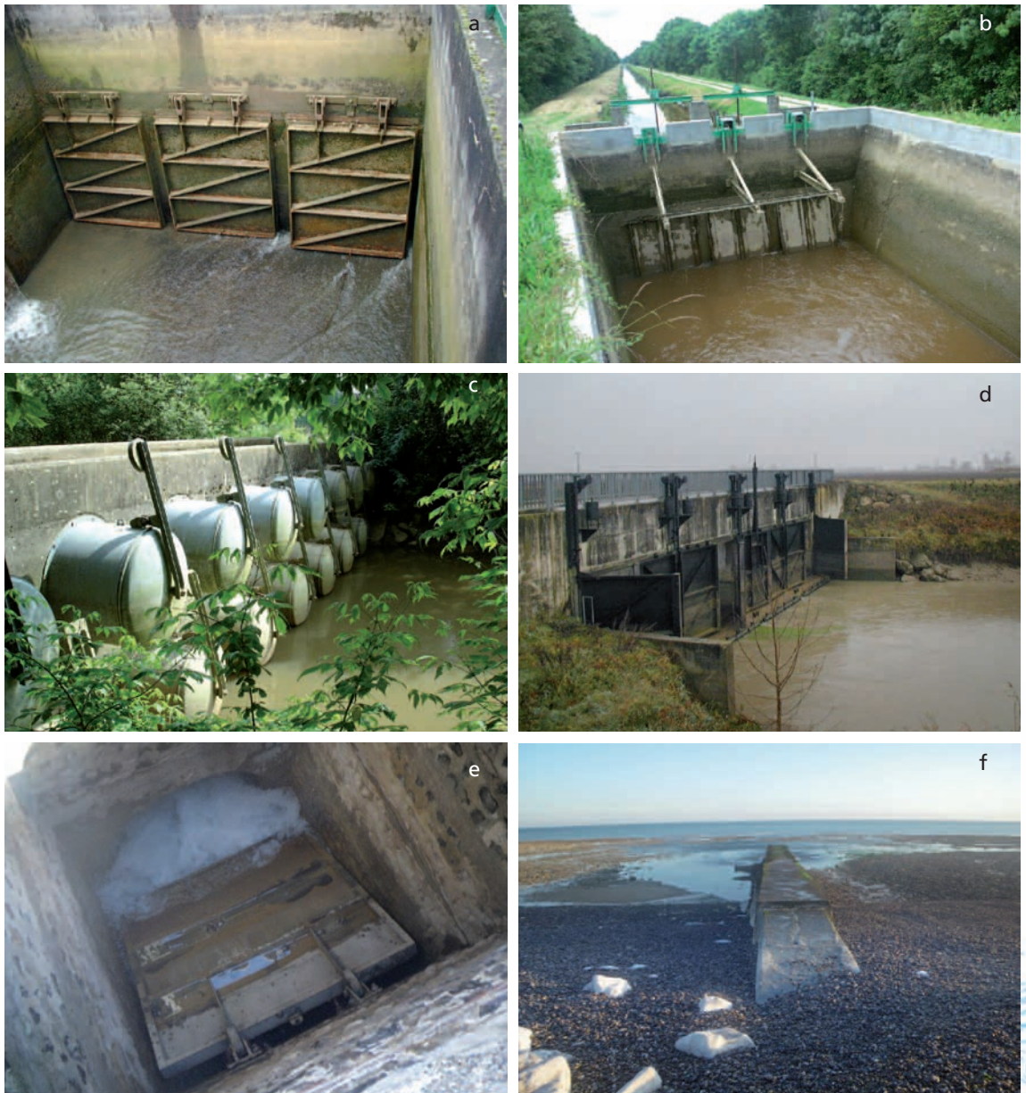
Examples of flap gates on tidal structures. (a) and (b) Flaps on the Médoc River, (c) "Stalin's organs" on the Arroudet stream, (d) structure comprising tide gates and flap gates in the lower section, on the Jale de Castelnaud River, (e and f) estuarine structure on the Yères River, comprising a flap gate upstream (photo on left) and a long culvert downstream (photo on right).
