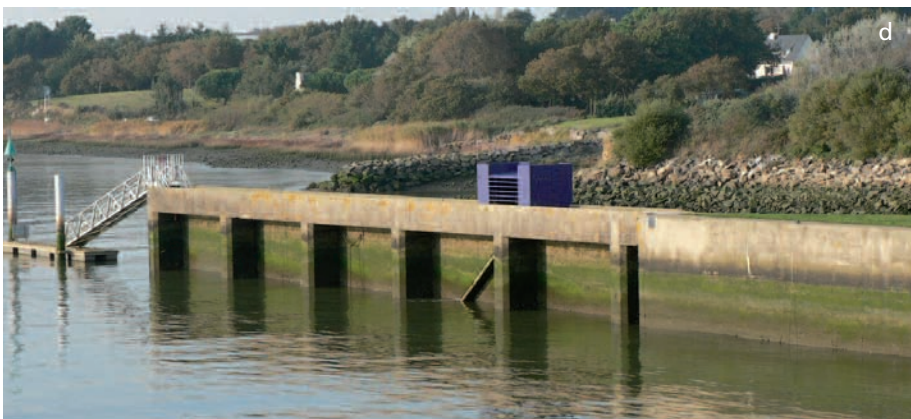
Examples of fish passes in estuaries. (a) and (b) Fish pass inside the Durdent estuarine structure, (c) and (d) fish pass for eels at the Arzal dam on the Vilaine River.
