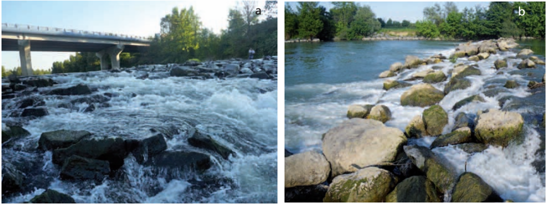
Examples of flows over rock weirs.
