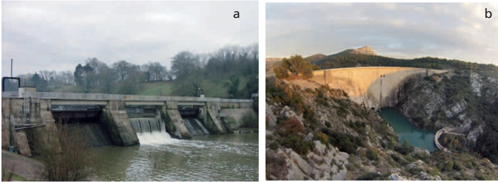
(a) Example of a gravity dam (dam storing drinking water in Apremont), (b) example of an arch dam (Bimont dam in the Bouches-du-Rhône department, 87 metres high).
