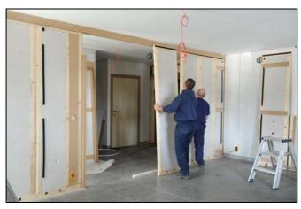
Figure 12. Mounting of interior wall (picture by courtesy of Atelier de l'Avenir)
