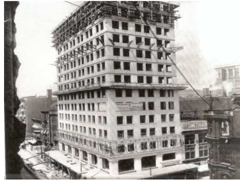
Figure 2. Ingalls Buildings, Cincinnati, Ohio, Elnzer & Anderson firm [9]
