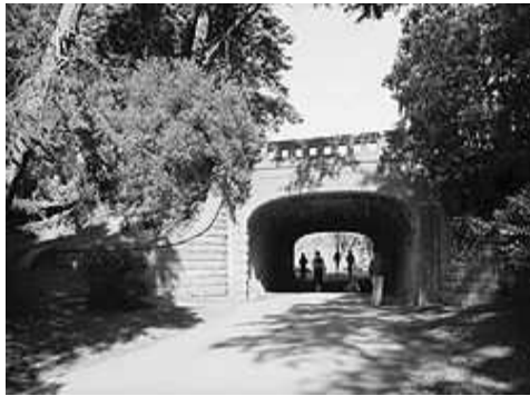
Figure 1. Alvord Lake Bridge by Ernest Ransome, [8]
