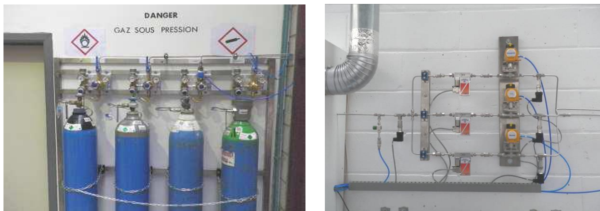
Figure 4.5: Bottle rack and gas supply
