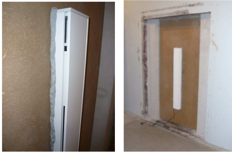
Figure V-33: Acoustic insulation measurement
