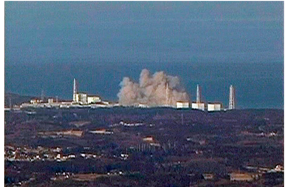
Fukushima nuclear power plant
