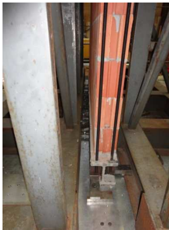
Figure 11 – View of the steel bars
