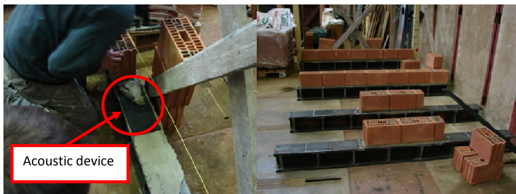
Figure 5 – Start of the wall construction
