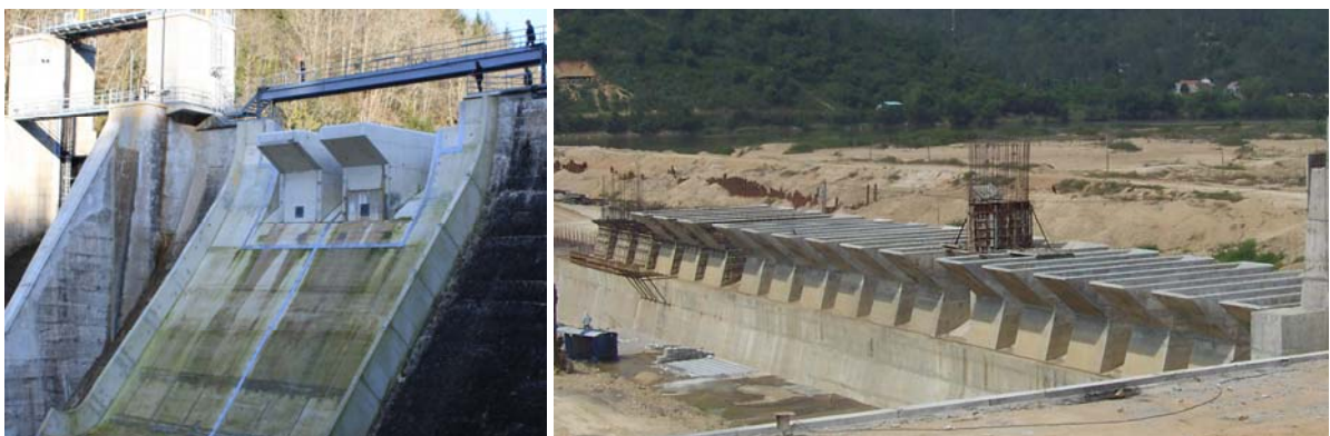
Figure 1 - PKW on the Etroit dam in France (left) and Van Phong PKW in Vietnam (right)
