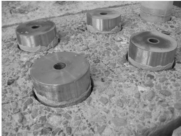
c) Dolly installation
