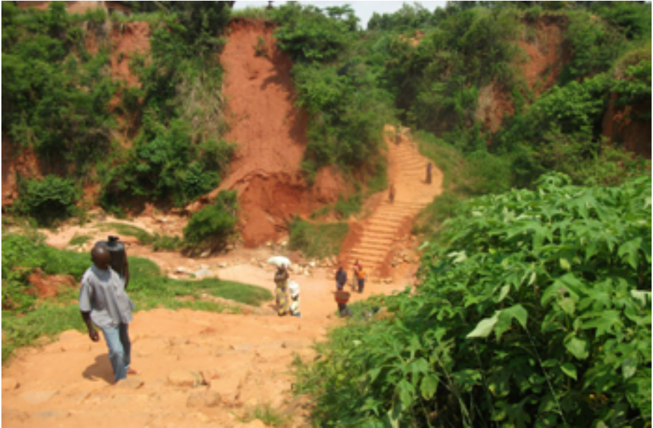
Figure 29 : Erosion de Mbala wa Tshitolo
