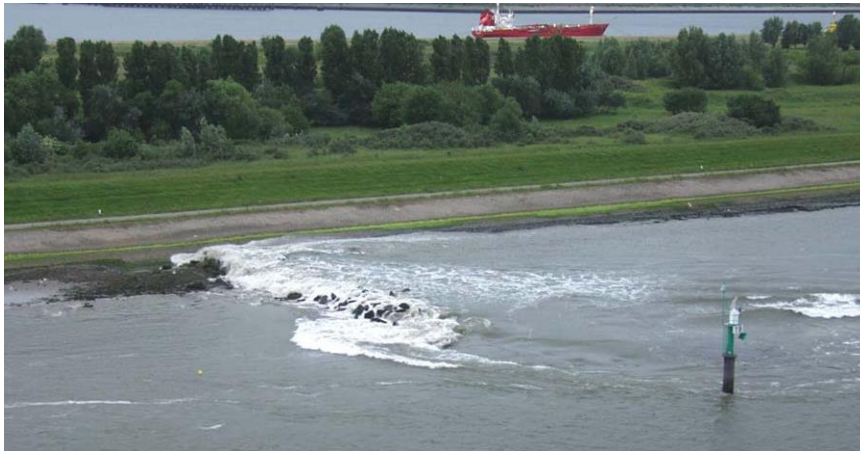
Fig. 1: Ship-induced waves overtopping a groin (photo: Uliczka, 2012)
