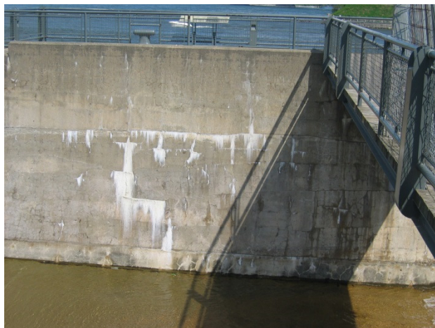
construction joints
