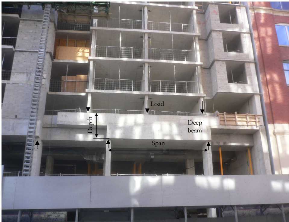
Figure 1.1 Transfer girder in a 15-storey building
