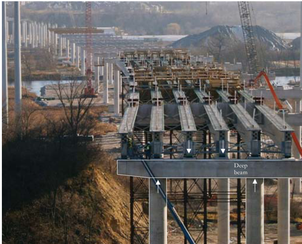
Figure 1.2 Cap beam in the substructure of a bridge
