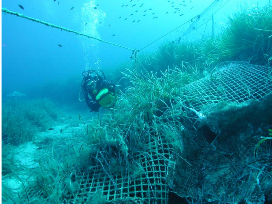
Fig. 8: Site supplemented with scour protection at the edges.
