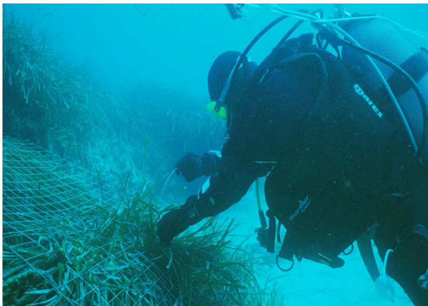
Fig. 3: Installation of the EAT grids over the dislodged parts of the Posidonia meadow.
